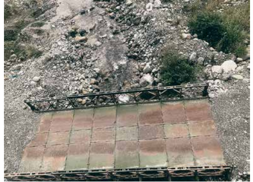
A makeshift crossing made of wooden planks under the Diffo bridge and a makeshift steel platform crossing under the Diffo bridge. Such platforms were regularly washed away during the monsoons, as the river streams swelled up.
