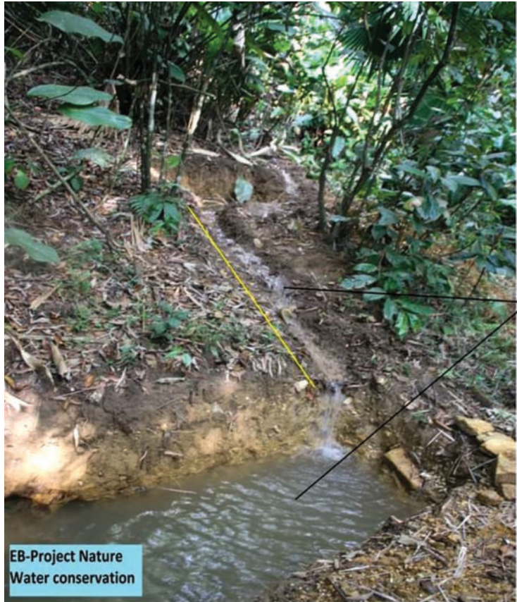
SIZE OF MASTER PIT : Any size depending on availability of space with depth 1.5 to 2 m. Master pit should be well protected.
