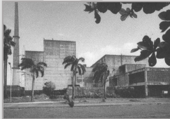
Tarapur Atomic Power Station
