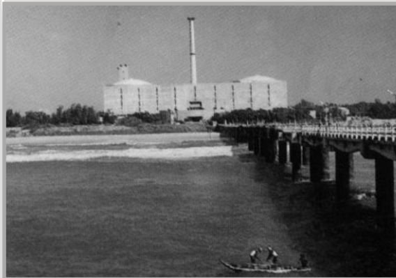
Madras Atomic Power Station (MAPS)
