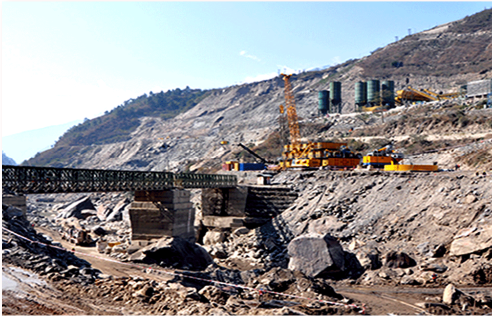
Construction of Punatsangchhu-I HEP, Bhutan
