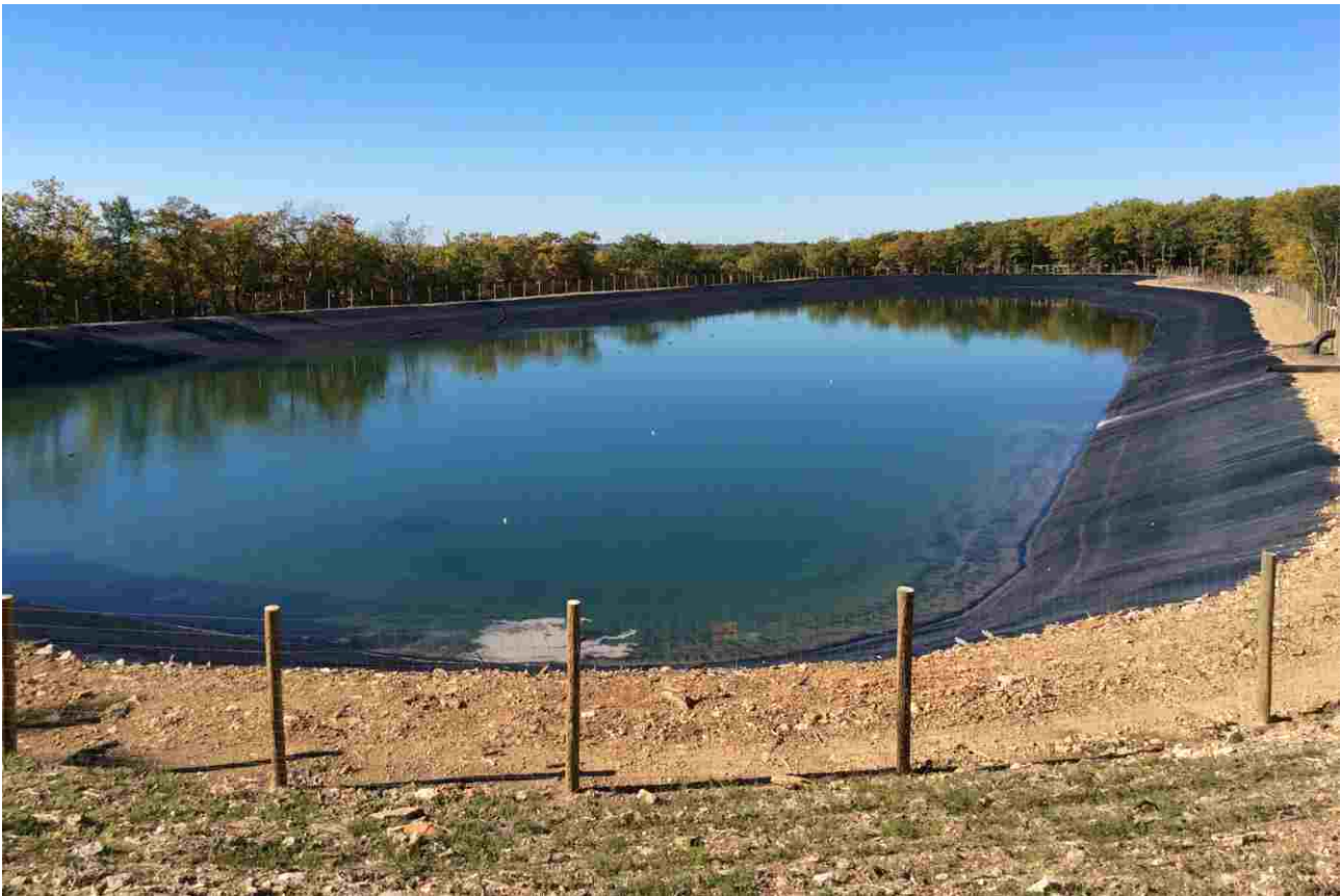
Freshwater Storage Pond at a Shale Gas Site in Pennsylvania
